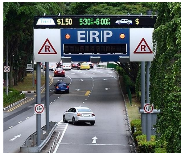
Figure 2-3 Electronic Road Pricing (ERP) gantry
