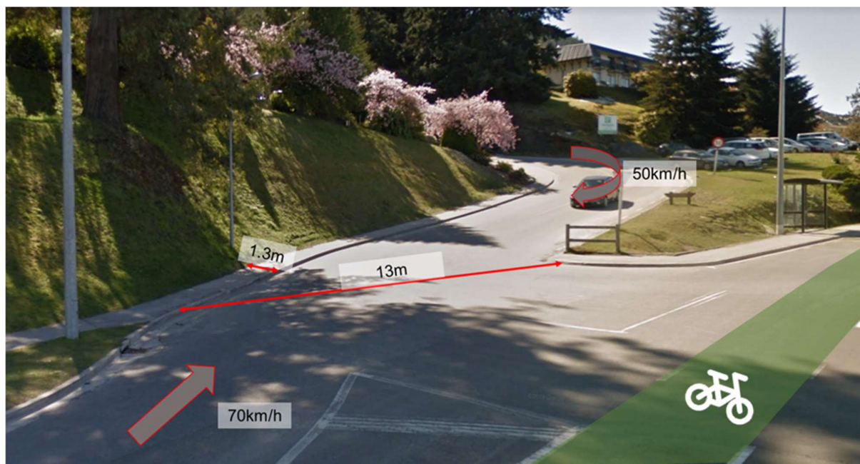
Figure 41: Inadequate Crossing Provision (Goldfield Heights/SH6A Intersection)
